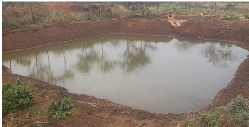
Figure 8. Pond construction for water harvesting in East Bale
